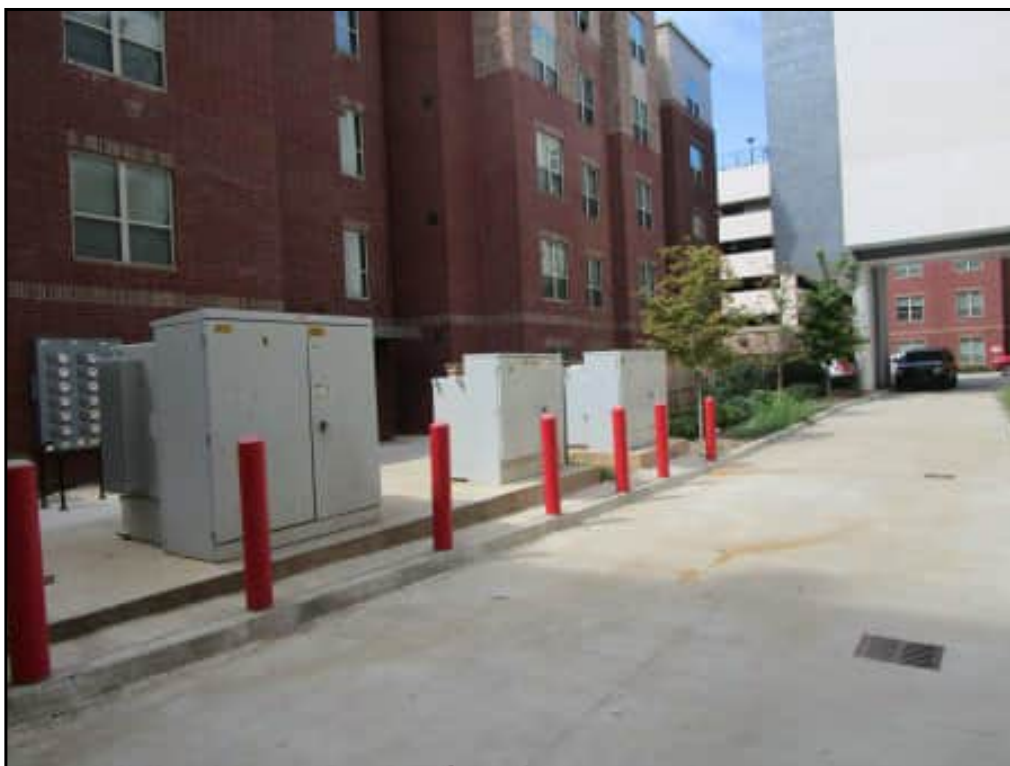
55 : Pad-mounted transformers
