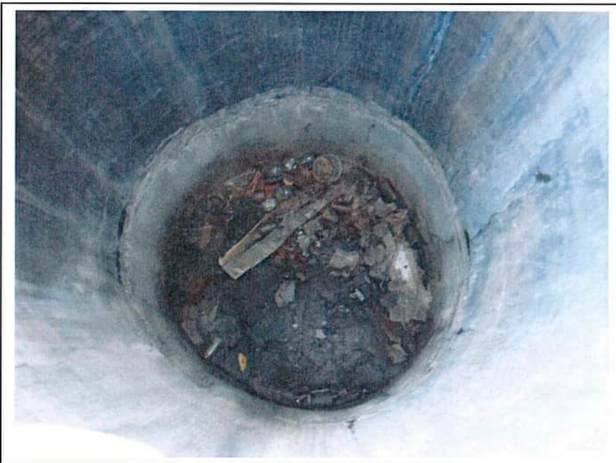
Photo 18. Bottom of rainwater collection cistern. Concrete lined brick.
