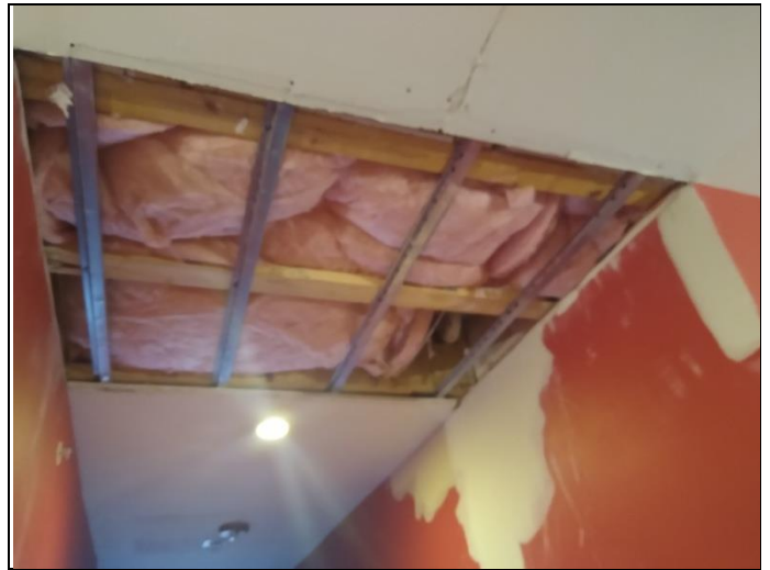
26. Water damage on hallway ceiling of basement
