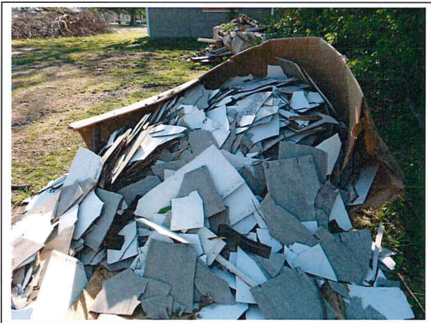
Photo 14. Non-friable asbestos exterior siding removed from structures.
