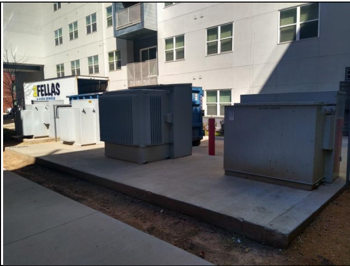
25. Pad-mounted transformers
