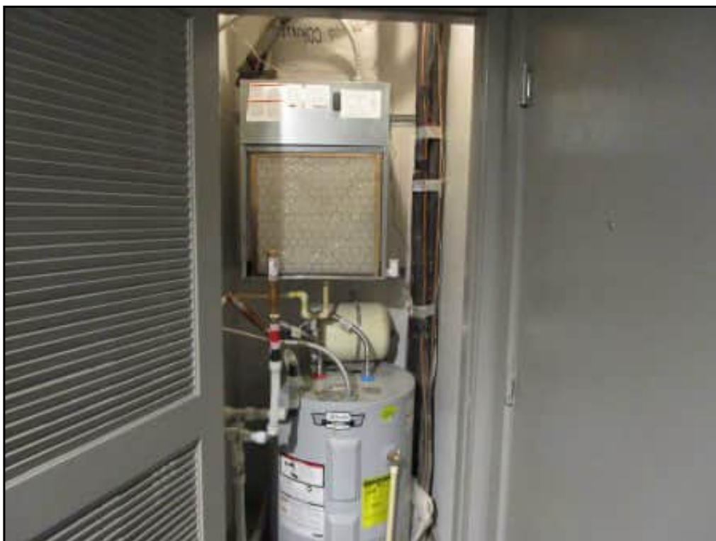
53 : Water heater and furnace
