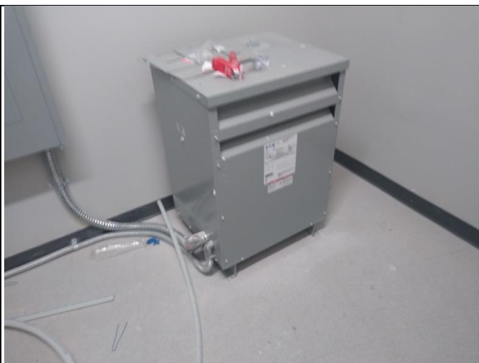
23. Interior dry-type transformer
